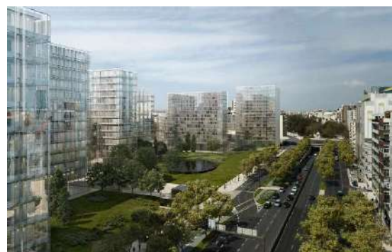
"ENTRECAMPOS" project — Lisbon, Portugal
