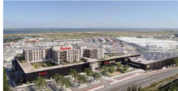
Alverca shopping centre transformation project — Portugal
