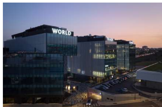
head offices of Leroy Merlin Portugal
